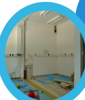
Dry Wall, Ceiling, Medical Gas pipes
